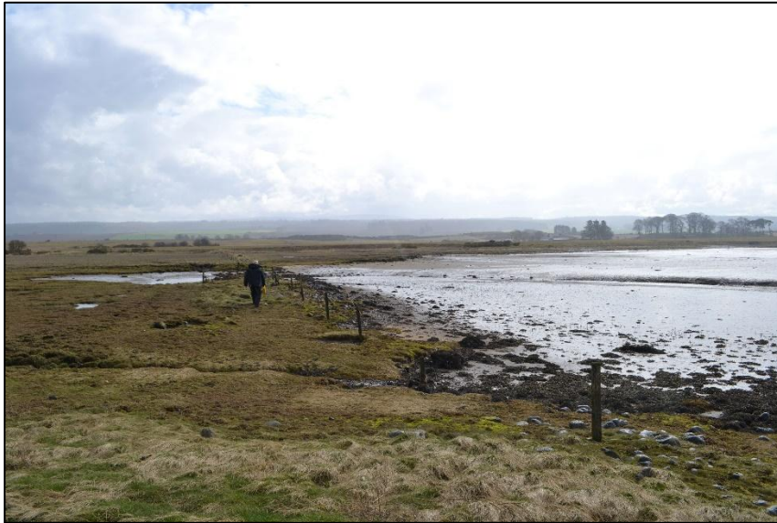
Figure 11 View of bulwark looking SE
