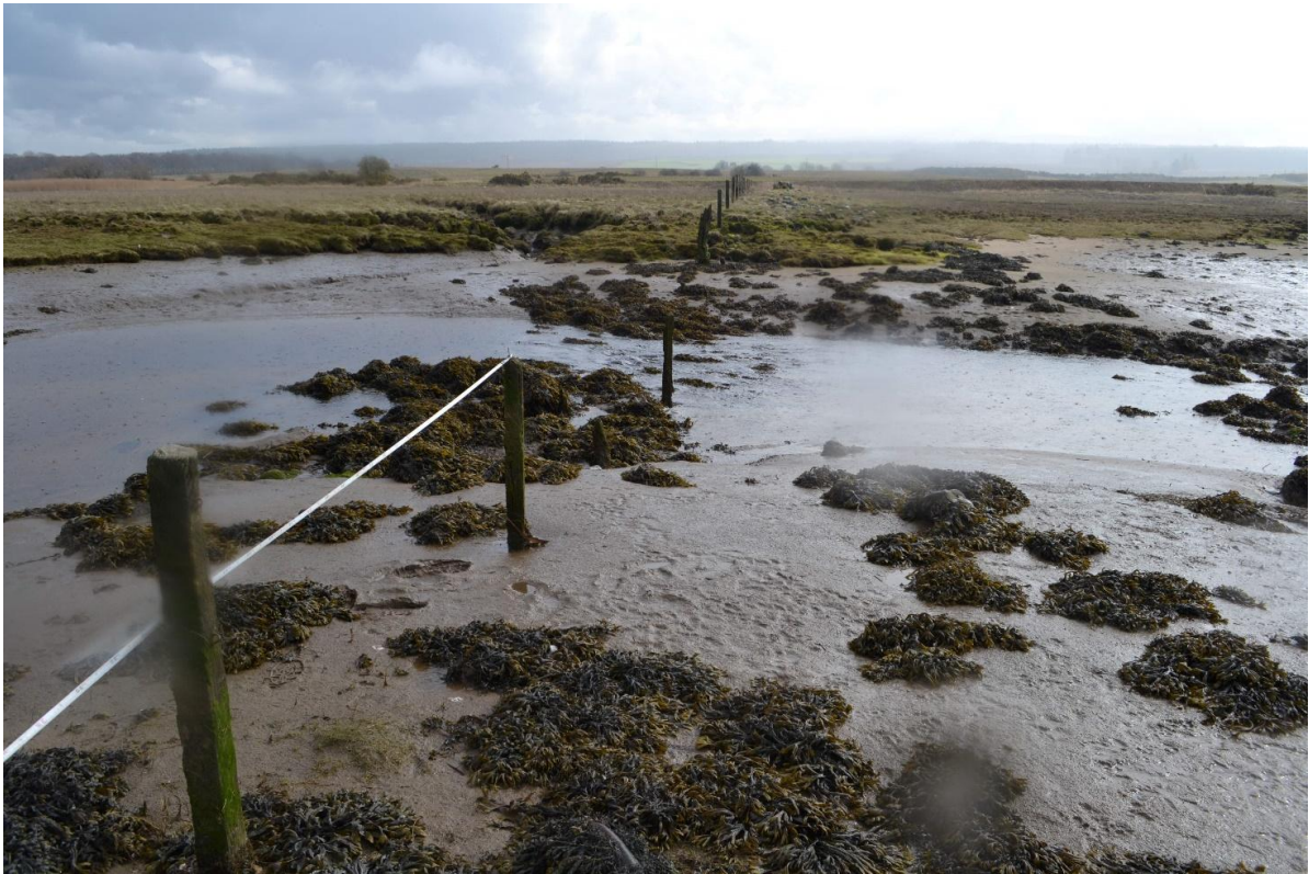
Figure 15 View of gap in bulwark with Rough Burn looking SE
